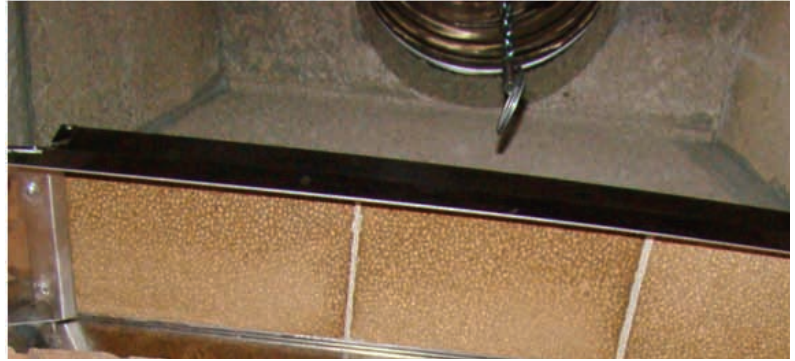
HearthCAT Installed in Isokern Fireplace.
