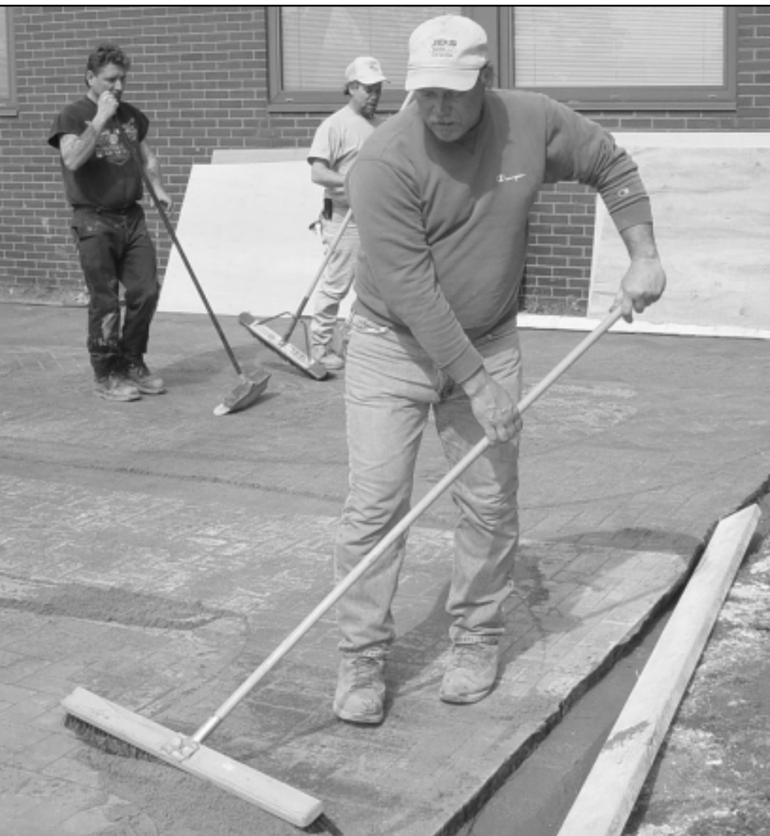
Figure 16: Sweeping Joint Sand
