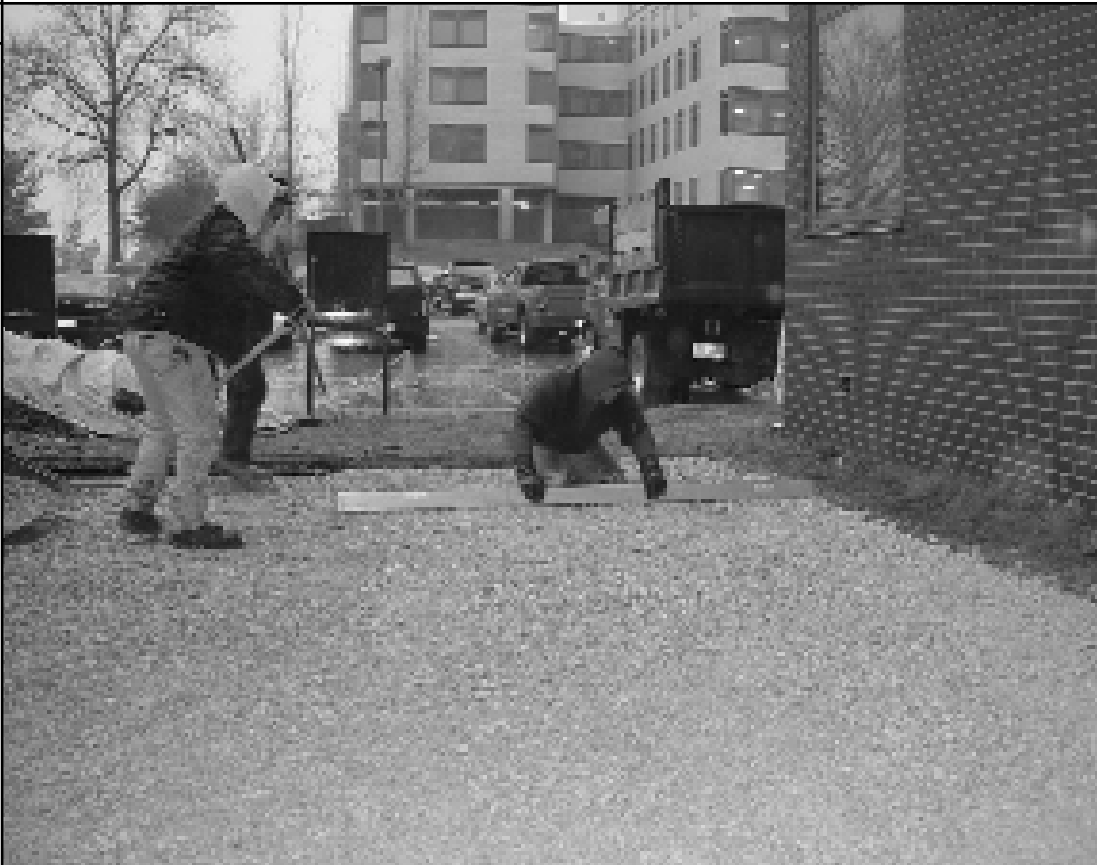
Figure 10: Leveling Base
