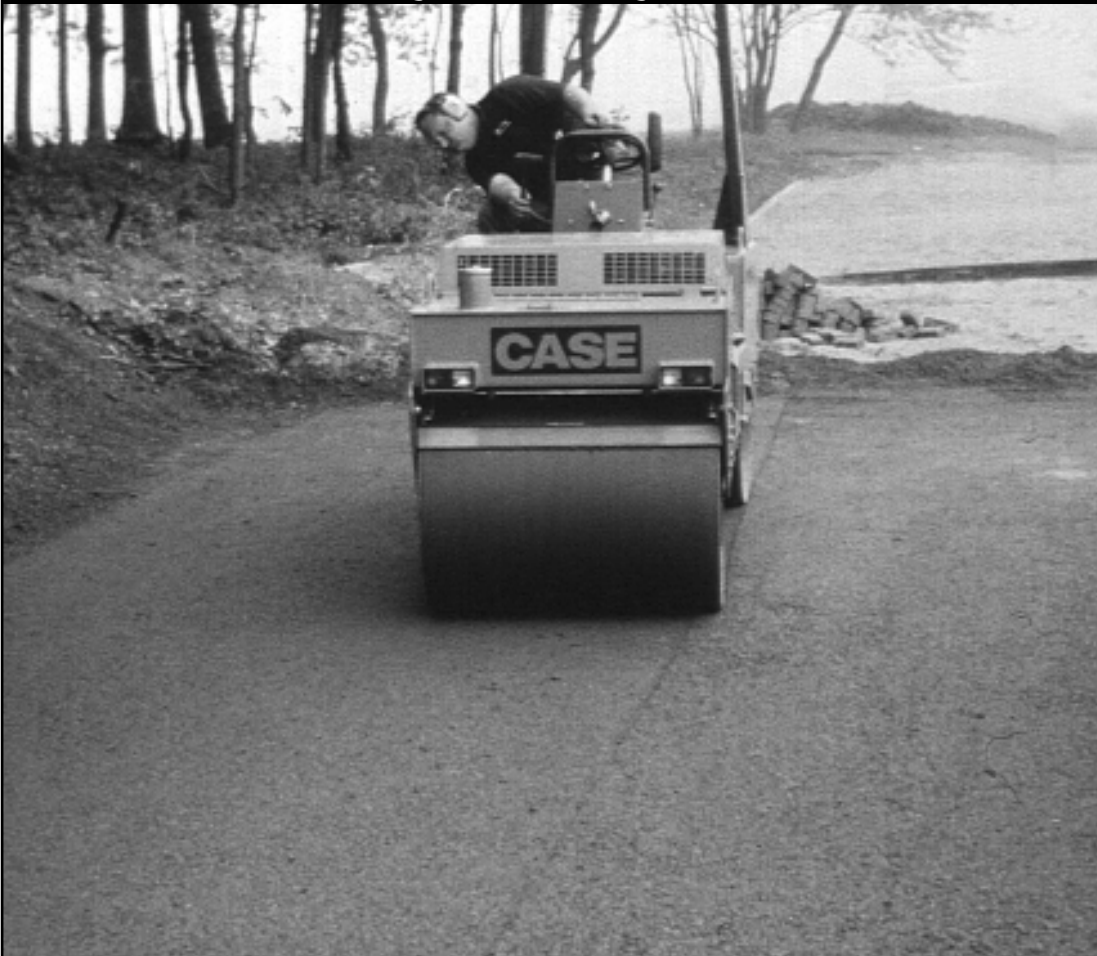
Figure 11: Proper Base Compaction
