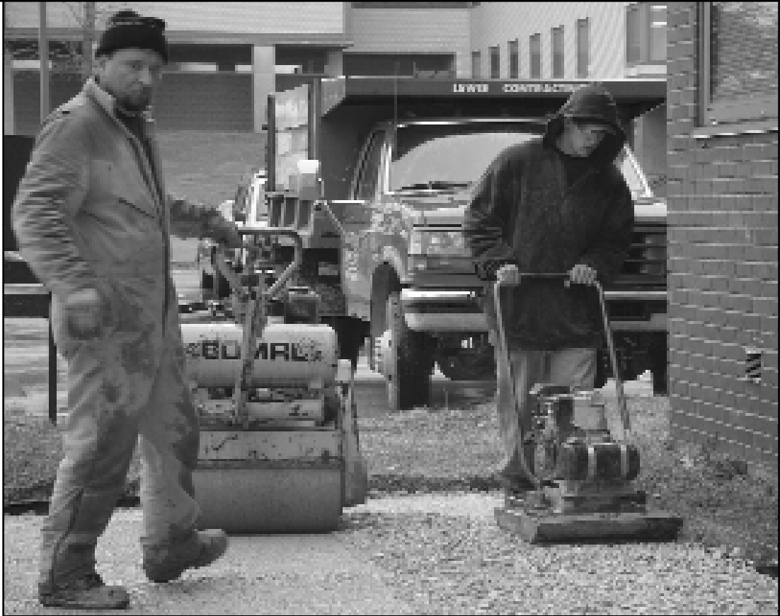
Figure 12: Compacting Near Edge
