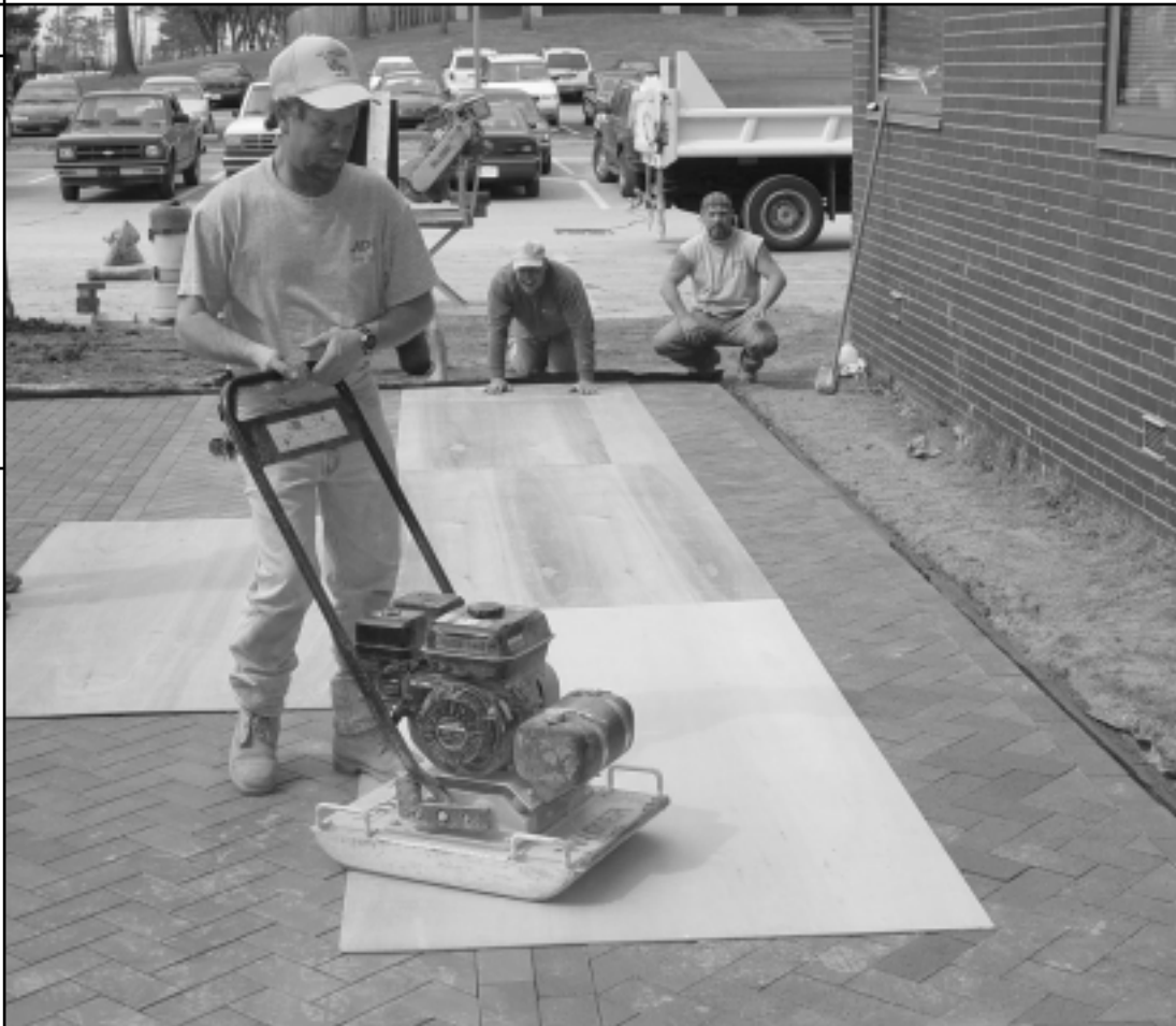
Figure 15: Compaction of Brick Pavers, with Protection
